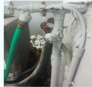
happens, you might have to call a plumber to install a new house valve and get your water running again. The picture on the right shows the house valve on the bottom. The valve on top is the hose spigot.
